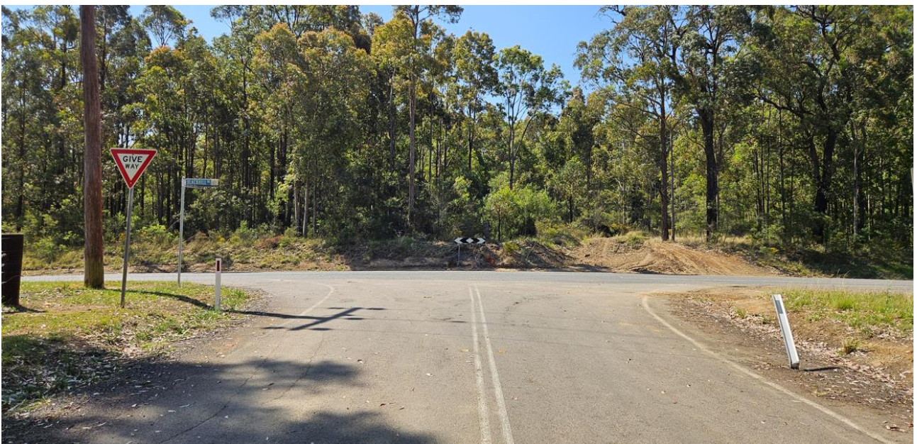
Plate 3.18 Existing signs and line marking at Black Hill Road/Browns Road intersection
