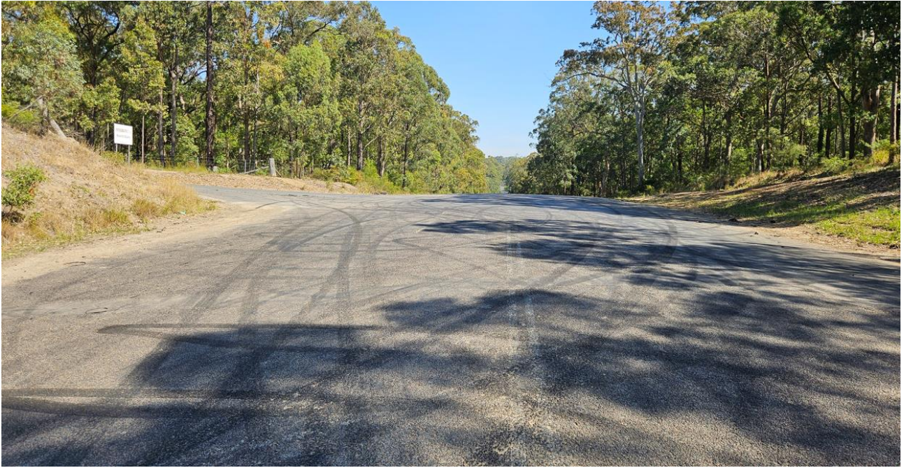
Plate 3.6 Existing faded centre line on Black Hill Road
