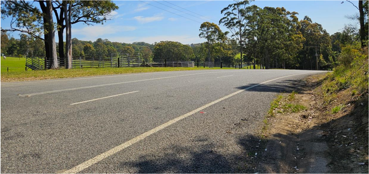
Plate 3.16 Shoulder widening on opposite side of Browns Road
