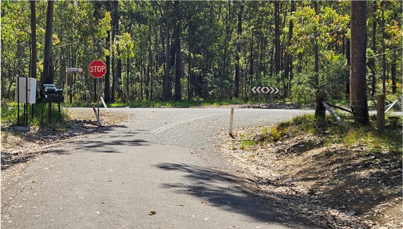
Plate 3.14 Existing signs and line marking at Black Hill Road/Meredith Road intersection
