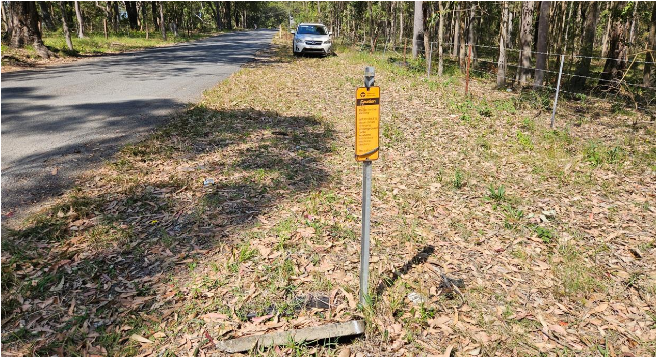
Plate 3.2 Utility services at the southwest corner of Black Hill Road/Quarry Access Road
